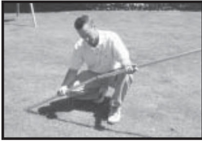
1- Slide upper poles onto lower pole and align the set screws holes.
